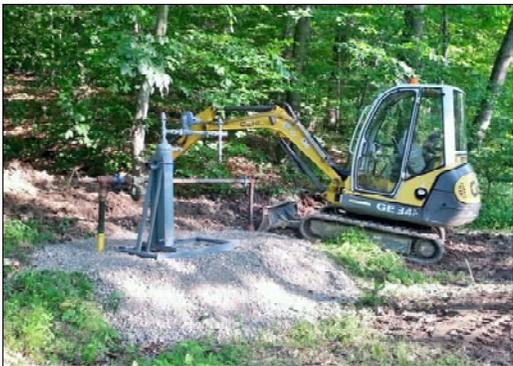
*A drip station and meter have been installed along the railroad bed as part of the camp's conversion to natural gas.*
